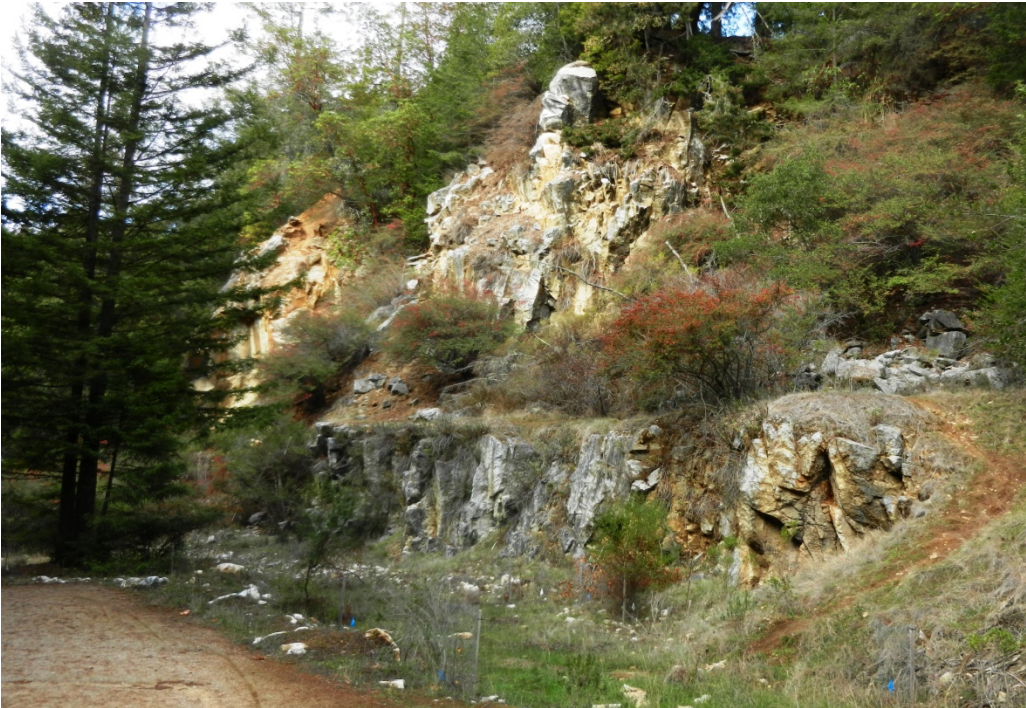
Figure 6. Close-up view of north rock slope behind stage area.
