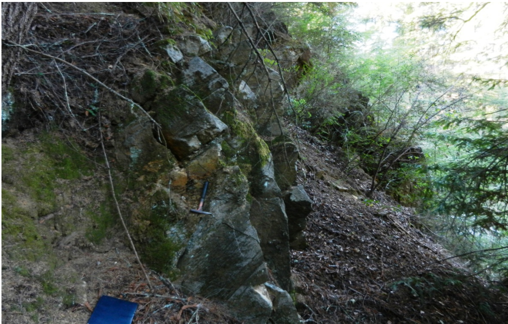
Figure 3. View of relic bedding/foliation dipping 40 degrees into slope at south rock slope
