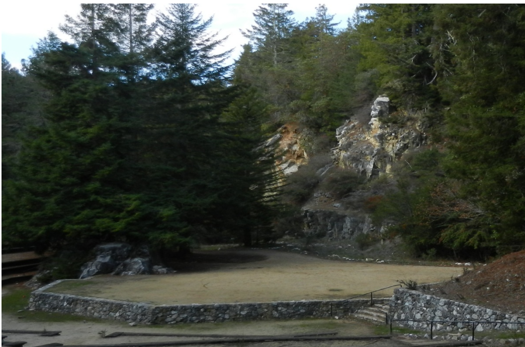
Figure 5. View of north rock slope behind stage area.
