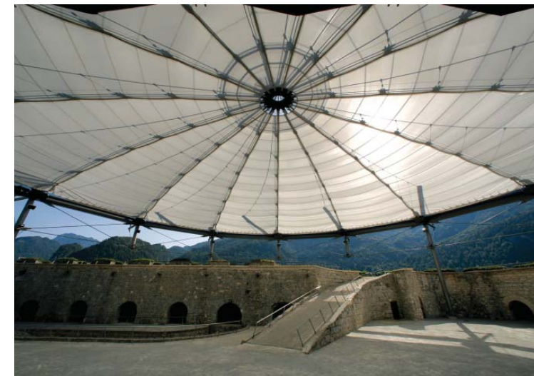
Tenara tensile structure
