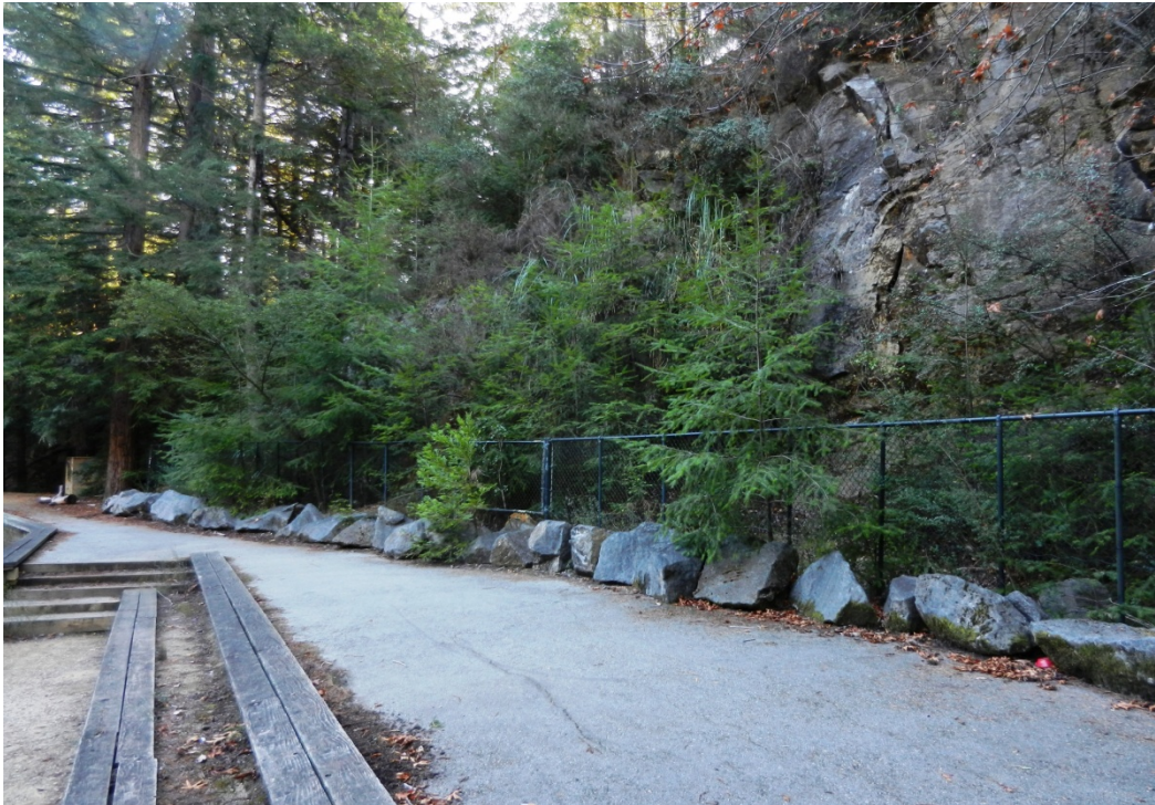
Figure 4. View marble rock slope south of seating area.
