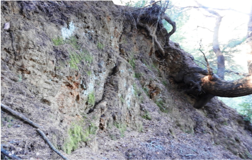
Figure 2. View of cliff formed in terrace deposits at top of south rock slope.
